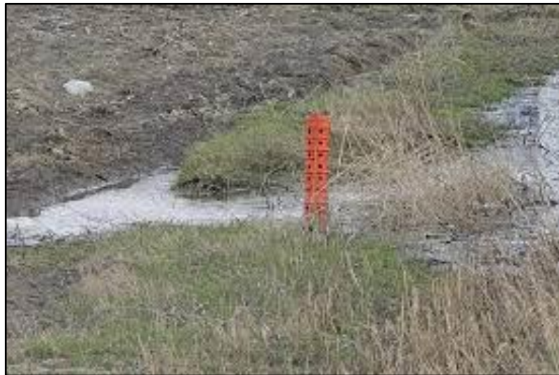
Figure 23. A view of a hickenbottom installed in an agricultural setting (Solenio 2021).
